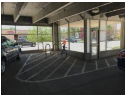
Finding 297249 Additional Photo
